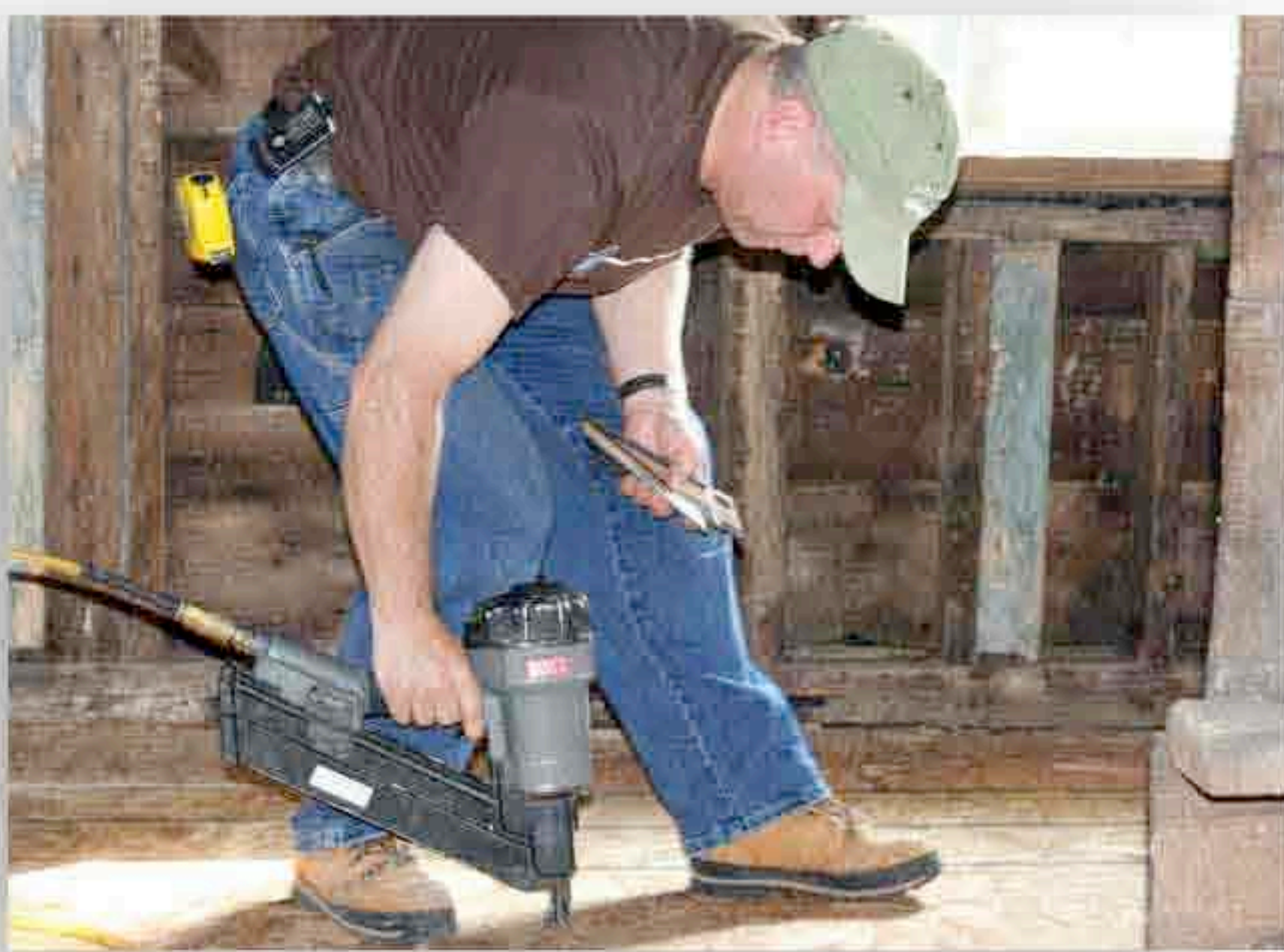
A volunteer installs sub-flooring for a mini-grant recipient
